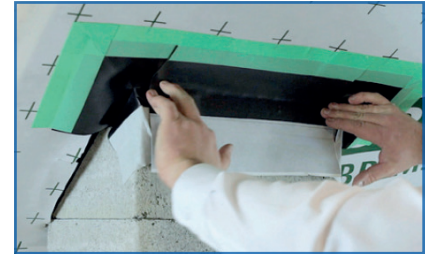
Inner corner can be plastered over
