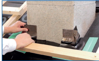
Inner corners plastering not possible
